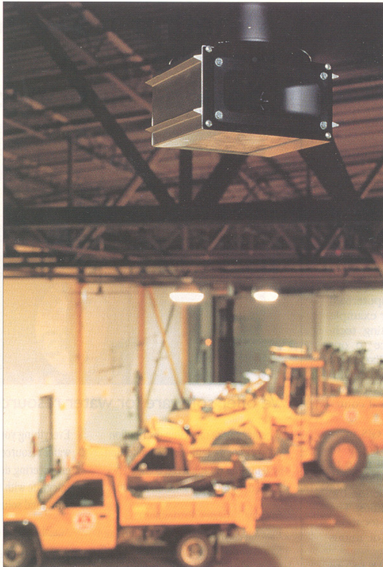
An ultrasonic unit solves the problem of pesky birds without endangering the health of the birds or employees.
